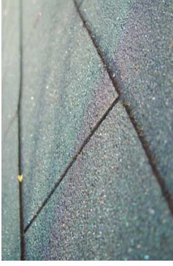
This image shows shingles that are in near perfect condition. Note that there is; no wear of granular, no waves in the surface, no layer underneath and no curling etc
