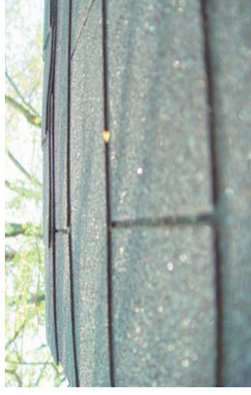
This image shows shingles that are in near perfect condition. Note that there is; no wear of granular, no waves in the surface, no layer underneath and no curling etc
