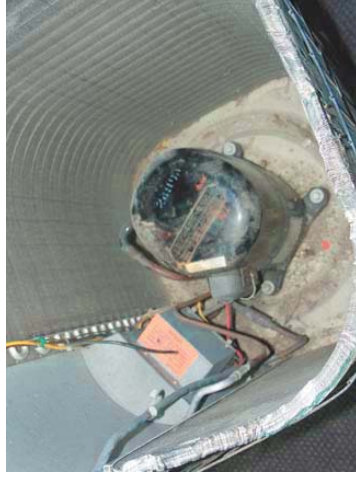
Inside this unit is the compressor. The compressor is the critical mechanical component.
